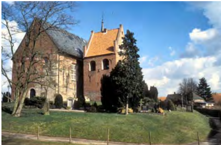
Figure 6: Church on dwelling mound, Zetel, Lower Saxony (Photo Henning Haßmann)
